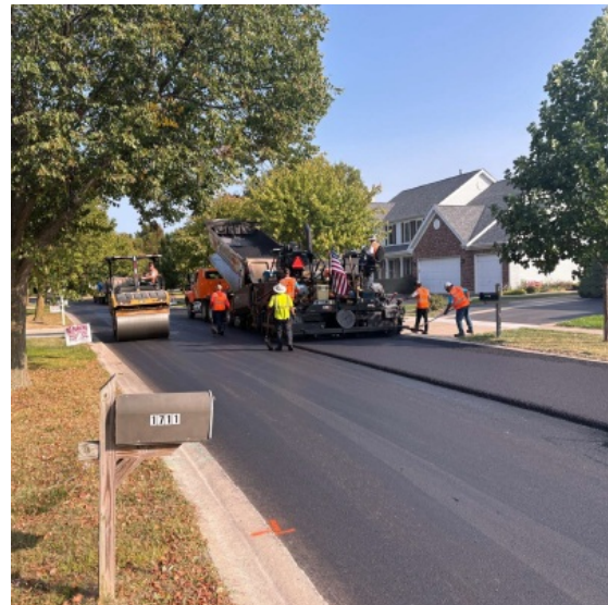
Paving the hot-mix asphalt surface course
